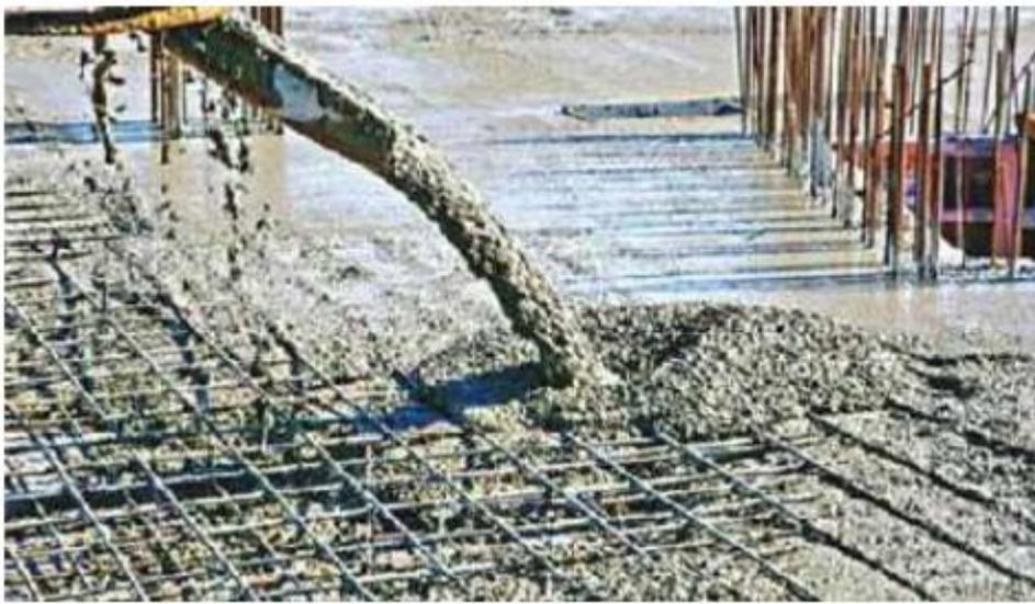
**Gambar 2.51 RCC (Reinforced Cement Concrete)**
